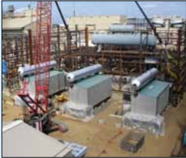
Installation in progress.
